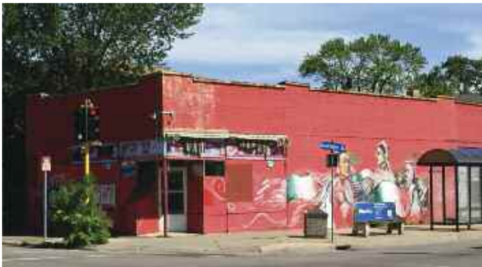
This building at 38th and Bloomington is scheduled to be demolished this summer due to structural and safety issues.
