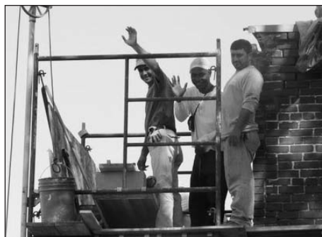
Joe Bailey and Rodak Construction up on the scaffolding.
